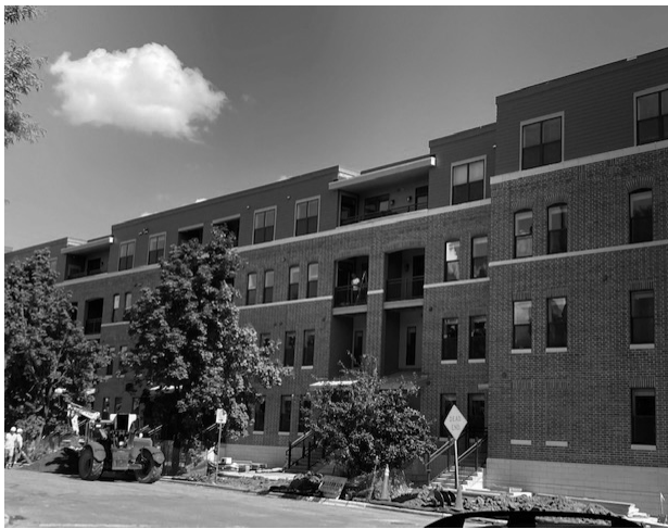
Fair Oaks Apartments, under construction
